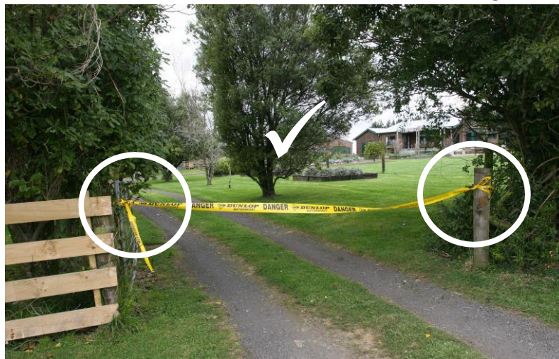
Figure 1 - Example of Correct Taping of an open Driveway (Ensure tape is pulled tight so it does not flap in the wind)
